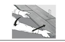
8. Tap end of plank with rubber mallet and tapping block to lock ends of planks together. Remove bridge and continue towards wall until installing the final plank in the row. Be sure to tap on edge of tapping block so as not to damage locking profile.
