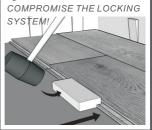
9. Use rubber mallet and pull bar to lock final piece in row. Insert spacer at end of row. Continue installation to final
